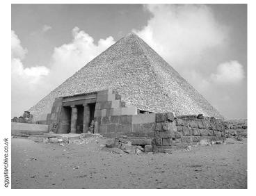
The Great Pyramid of Khufu, built 4500 years ago, is one of the world's largest structures. It is estimated to have taken 100,000 men over 25 years to build using 2.3 million blocks averaging 2.5 tons each. The blocks ranged from 2 to 15 tons. The pyramid sits on 13.5 acres of land, is 756 feet square at its base and 480 feet tall.
